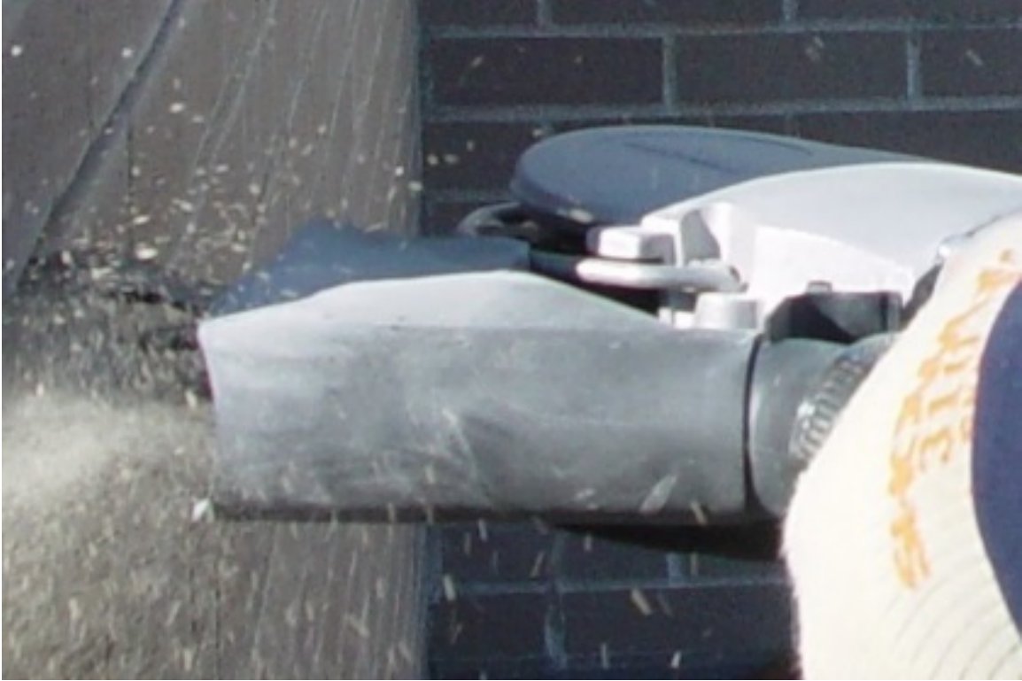
Figure 2 - Dust extraction hood in use (NIOSH photo)
