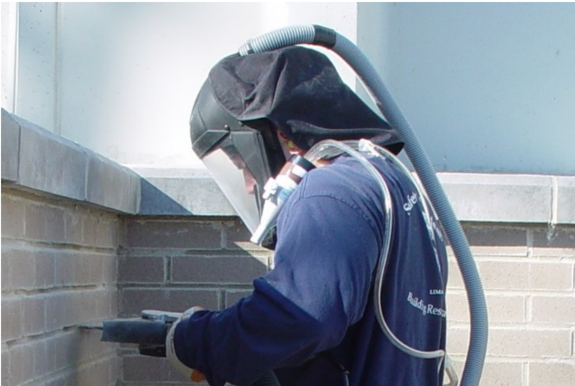
Figure 4 – Cyclone sampler in the breathing zone (NIOSH photo)
