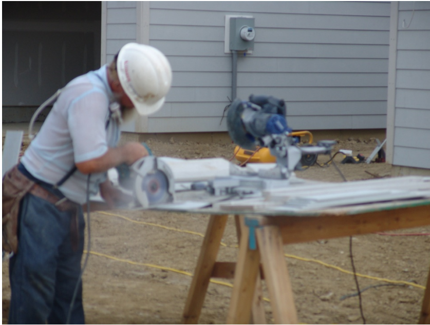
Figure 2 – Laborer (cutter) operating a circular saw and cutting the fiber-cement siding.
