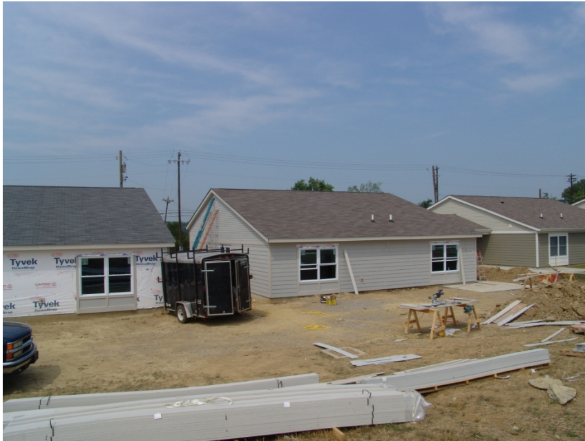
Figure 1 – The Construction Site.
