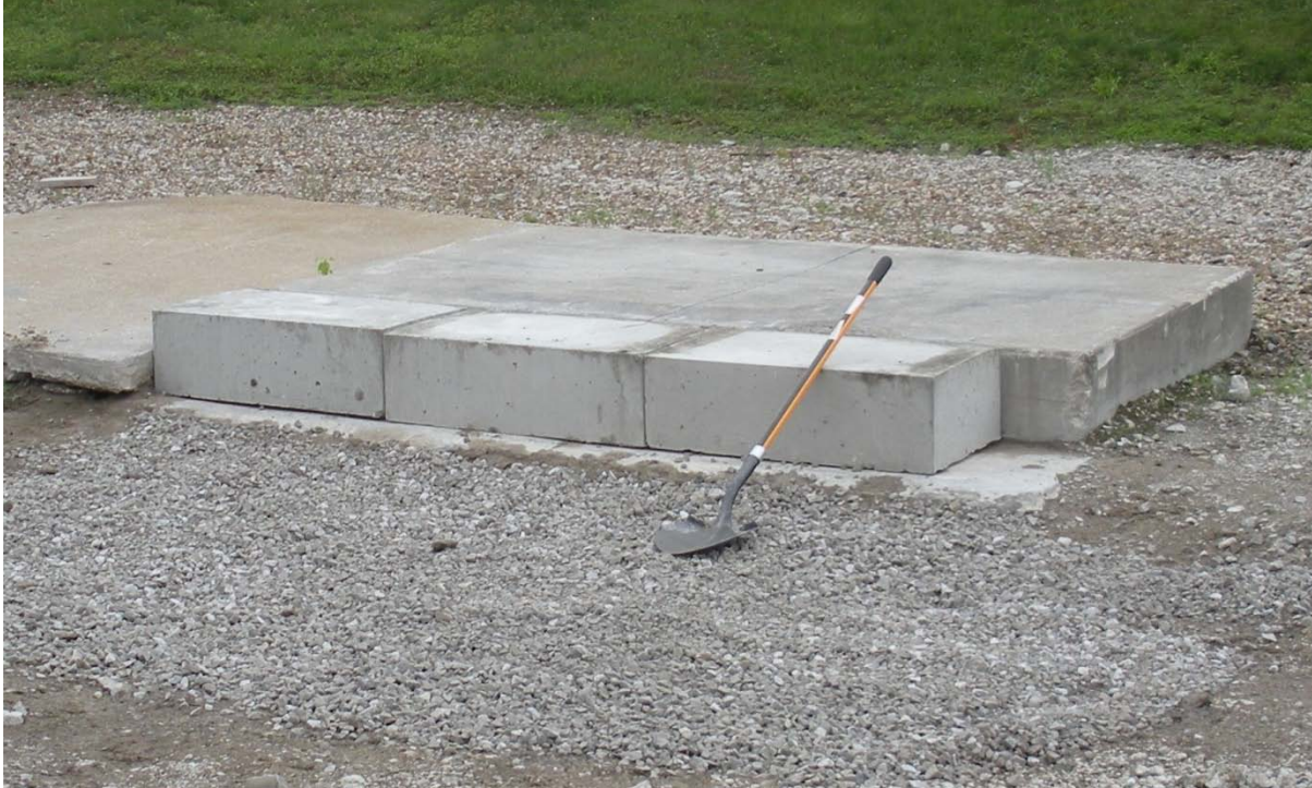
Figure 2 - Holes Were Drilled in Three Solid Concrete Blocks Placed in Front of a Concrete Slab
