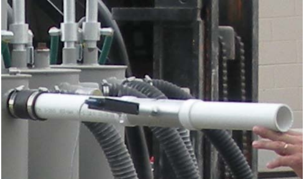
Figure 6 - Measuring Air Flow at the Dust Collector
