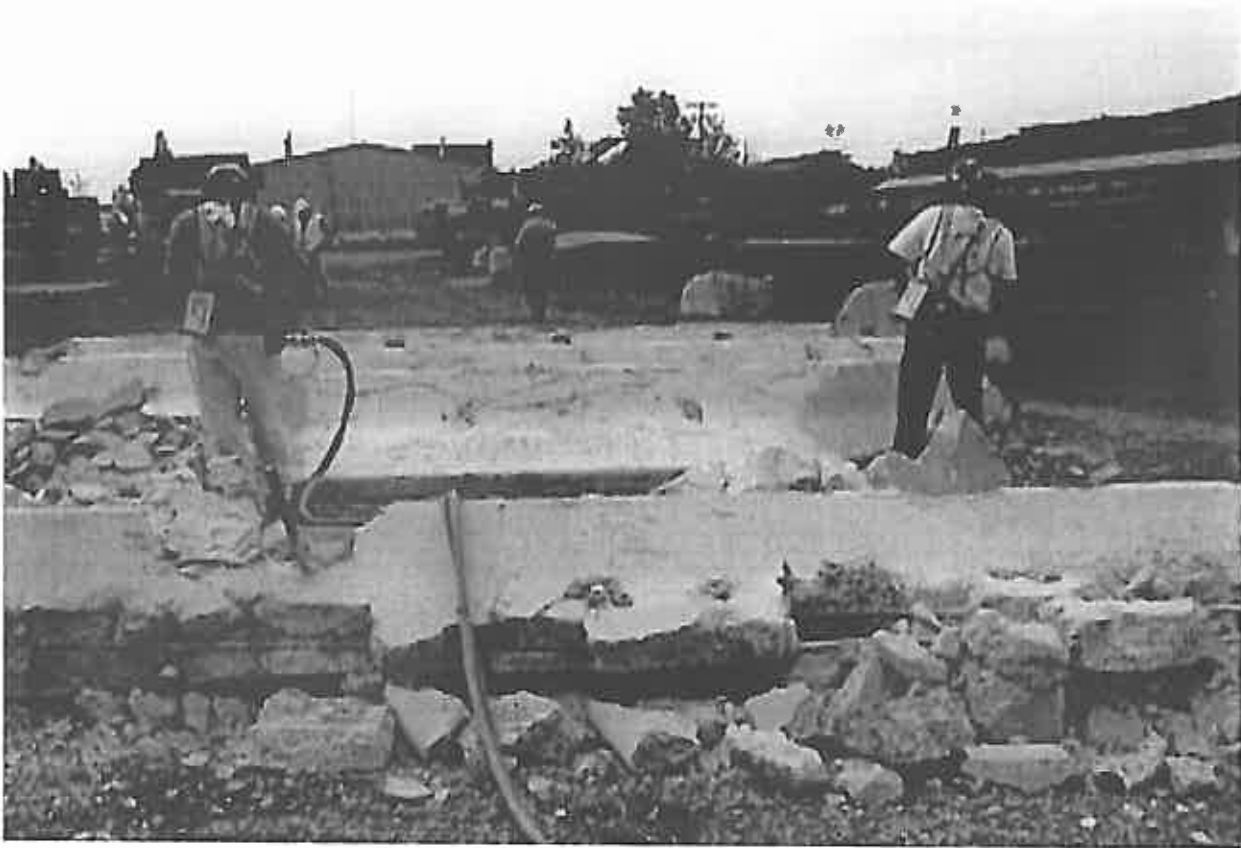
Figure 5: Workers during a wet trial.
