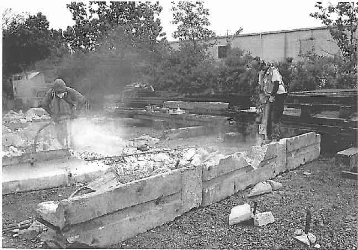
Figure 6: Workers during a dry trial.
