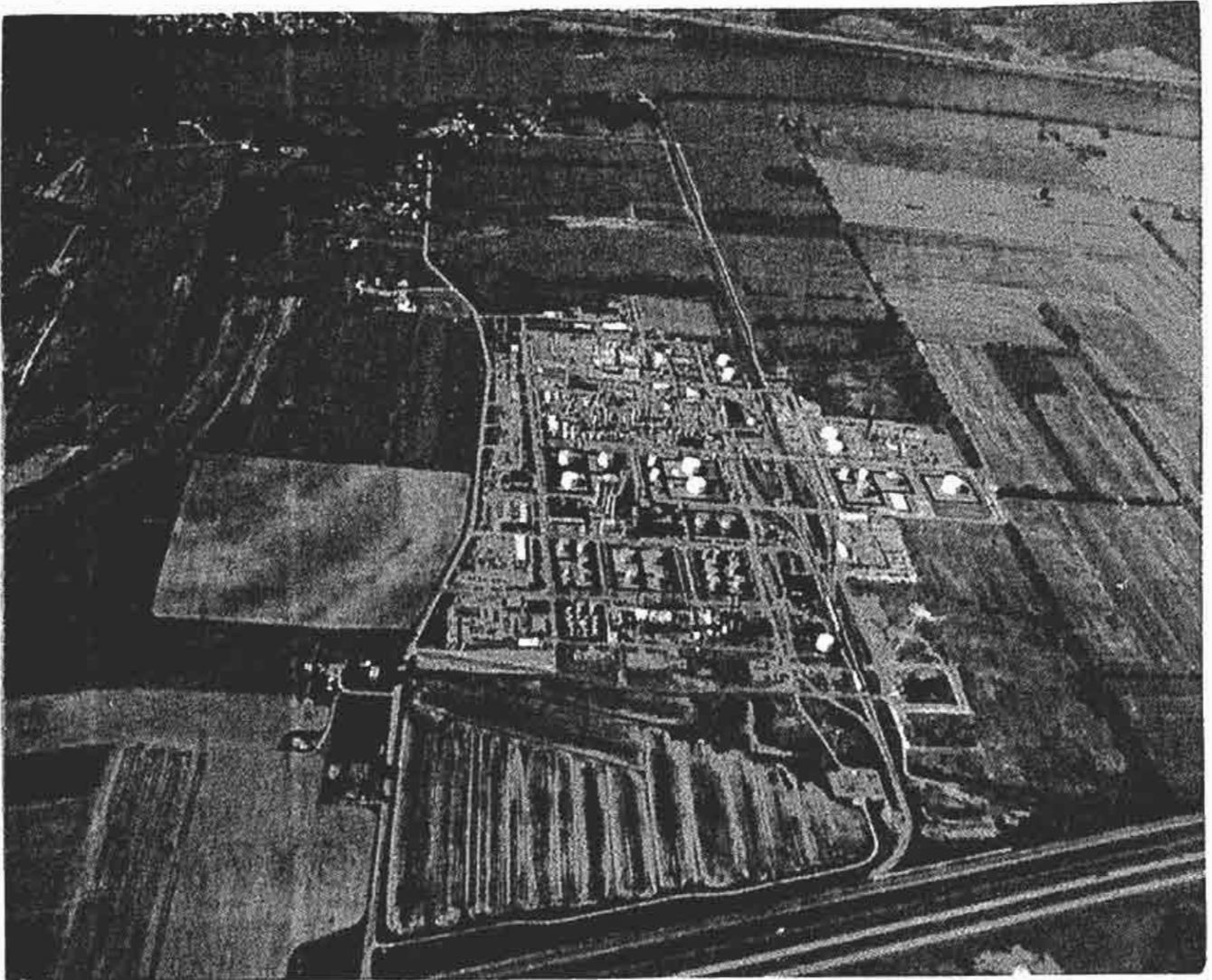
Figure 1. Haverhill Site (Haverhill, Ohio - on Ohio River) USS Chemicals Division U.S. Steel Corporation
