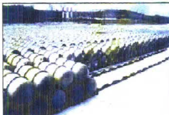
Figure 14. Concrete-floor storage yard for depleted uranium UF 6 cylinders at the Portsmouth, Ohio enrichment plant.
