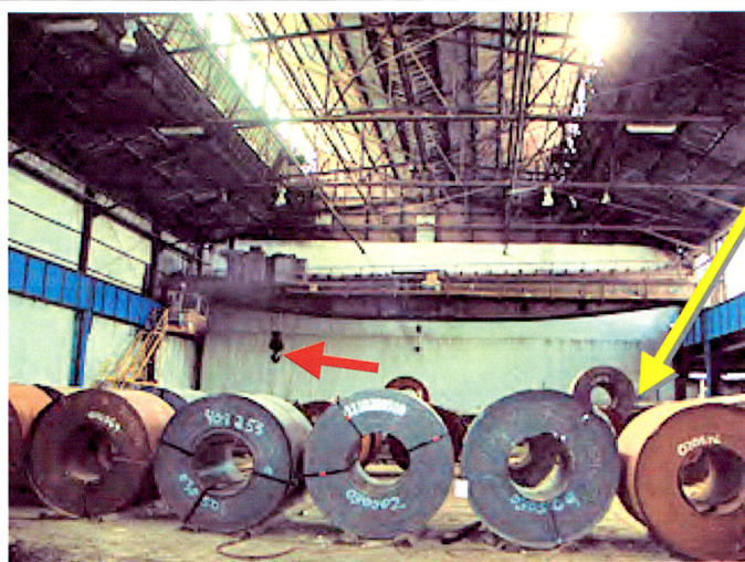
LEGEND. Gondola/cab far left hangs below crane. Catwalk above and hanging hook (arrow) blocks measured Co-60 radiation.
