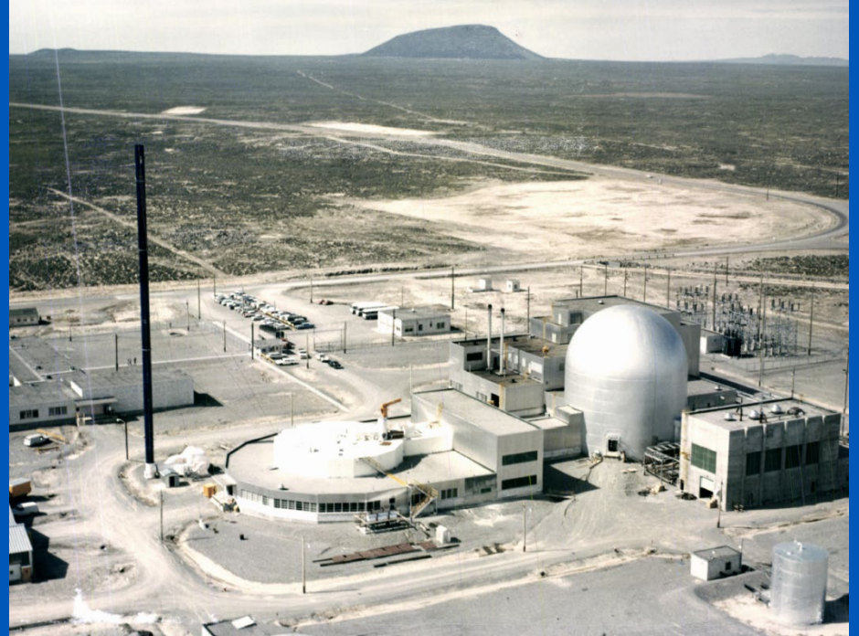
Aerial Photo of the EBR-II Complex
