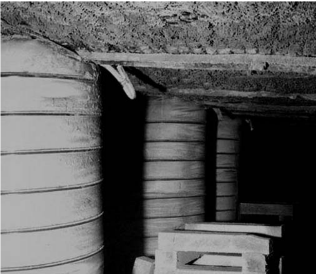
Figure 2 — Pumpable roof support in longwall tailgate showing how the support can achieve full contact with mine roof.
