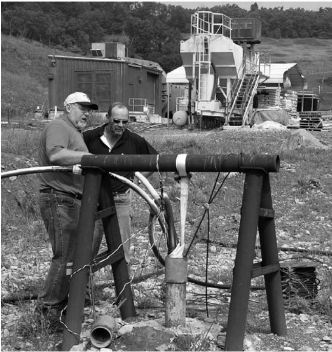
Figure 19 —Cement slurries are pumped down the borehole in separate lines (pump mixing station in background).
