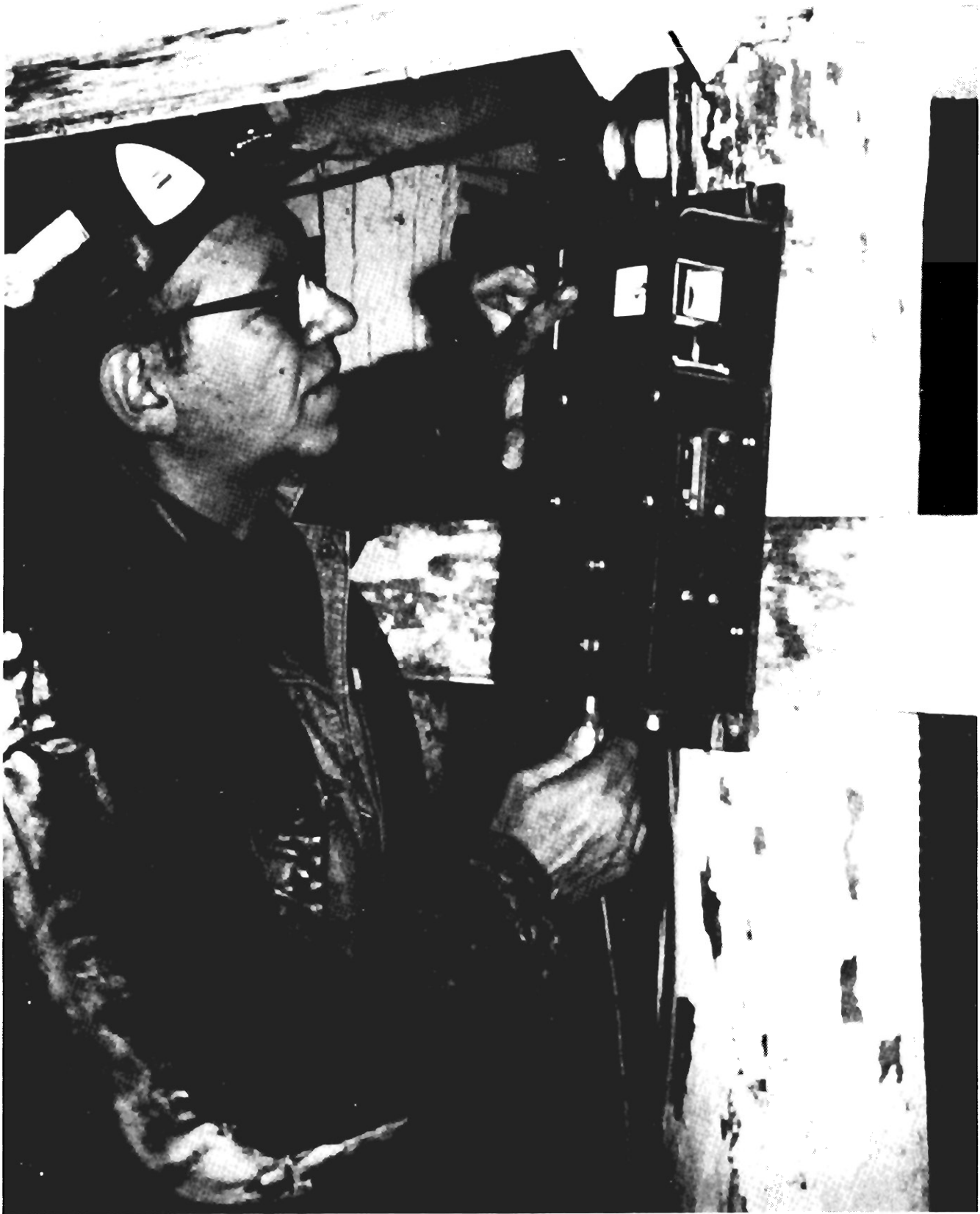
Figure 5-30. Three-Function Environmental Monitor Installation.
