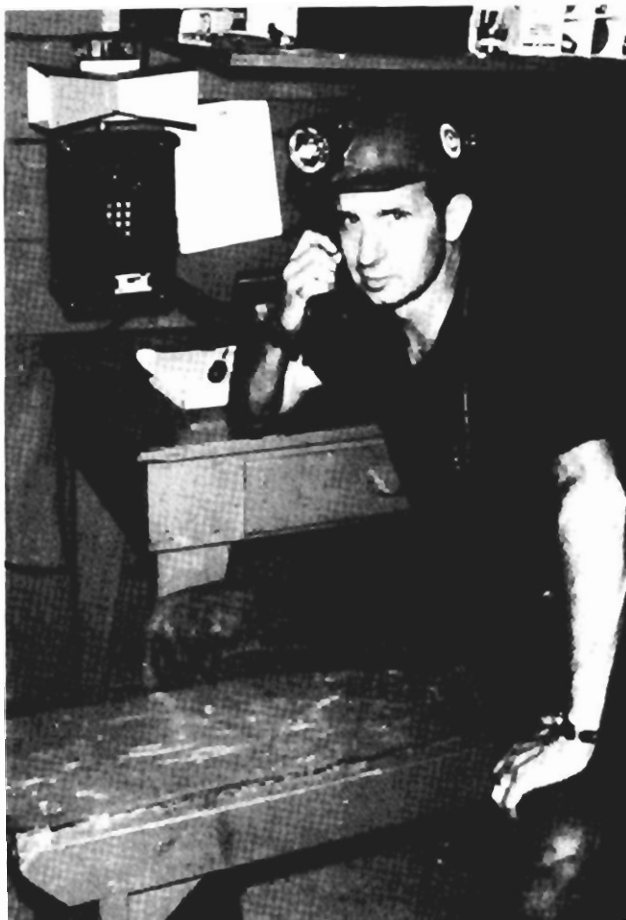
Figure 4-28. Underground Electric Shop Telephone Installation.
