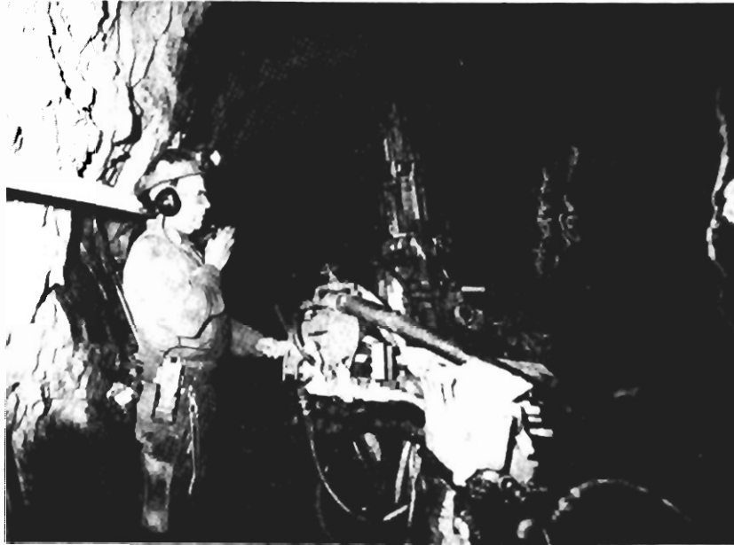
Figure 5-27. Fan-Hole Drill Operator With Noise-Reducing Speaker-Microphone and Belt-Suspended Radio.
