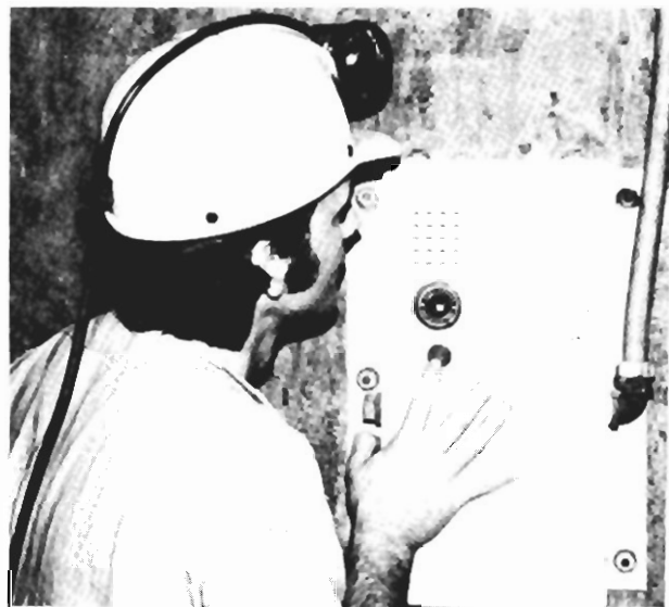
Figure 4-5. Cage Installation at Sunshine Mine.
