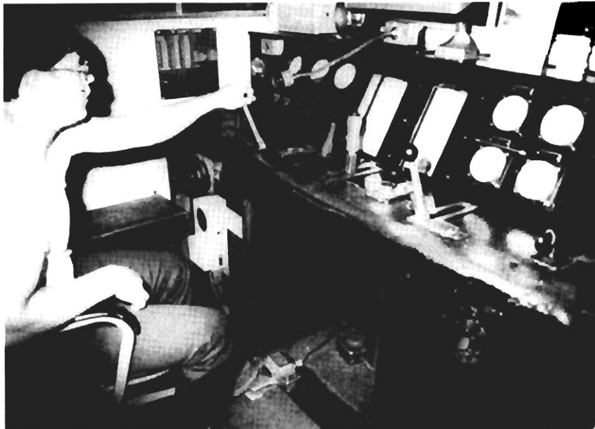
Figure 5-9. Hoist Operator's Equipment.
