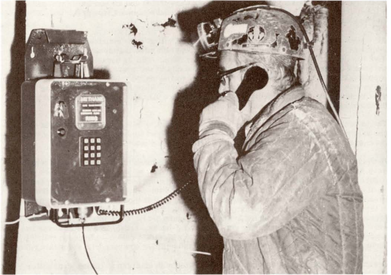
Figure 5-28. Underground Telephone Mounted on Wooden Post.
