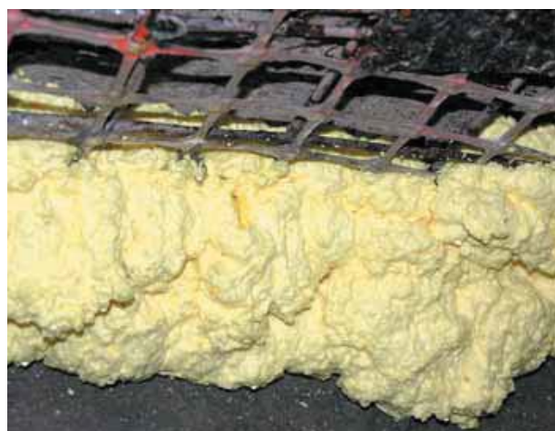
Figure 4. Polyurethane foam sealing stopping at roof on pressurised stopping side for Test 3
