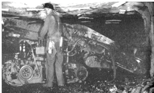
Figure 14. Machine loading with roof bolts.
