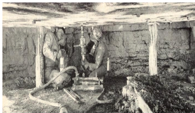
Figure 10. Installing roof bolts with a hand-held stopper drill.
