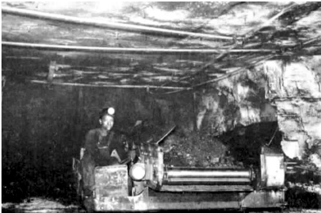
Figure 13. Shuttle car haulage with roof bolts.
