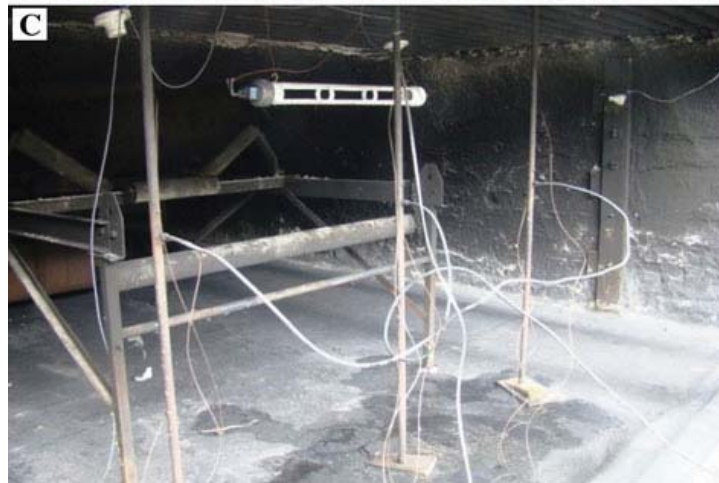
Figure 1. Photographs showing the fire suppression facility (a), the rubblized coal with strip heaters and conveyor belt (b), and the gas sampling and other instrumentation at the exit of the fire suppression facility (c).
