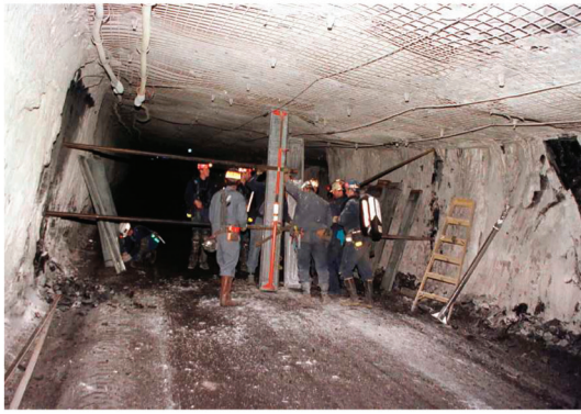
Figure 4 — Construction of a Kennedy steel panel stopping in the No. 2 entry.
