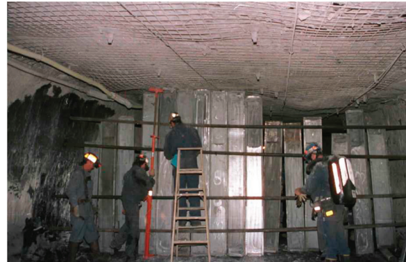
Figure 4 — Construction of a Kennedy steel panel stopping in the No. 2 entry.
