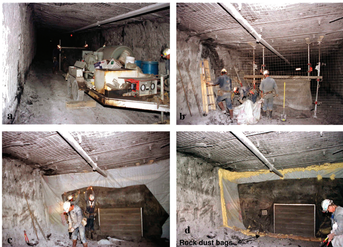
Figure 3 — A partition being built for the foam generator.
