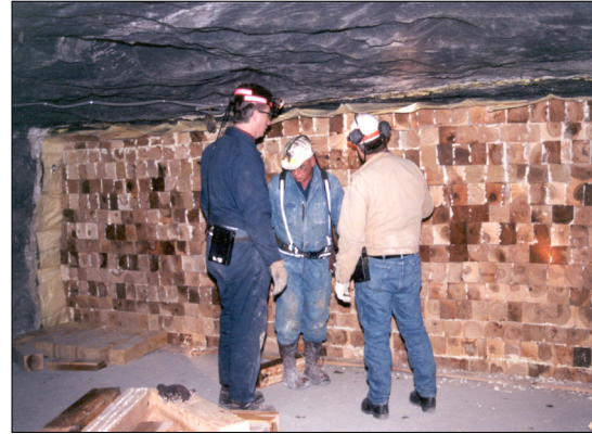
Figure 3- Pre-loaded wood crib seal
