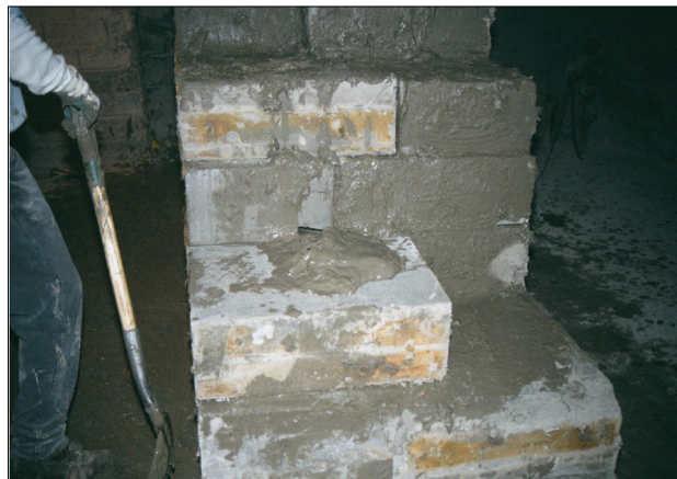
Figure 6 - Omega seal construction
