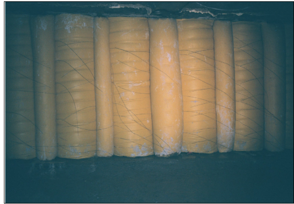
Figure 8 - Completed HeiTech seal
