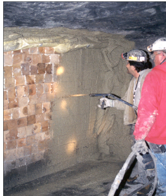
Figure 4- Coating wood seal with Strata sealant
