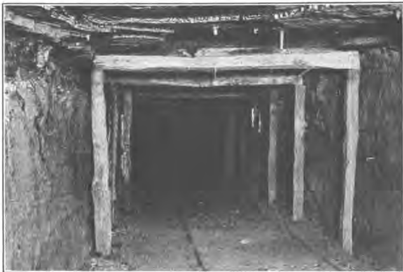
FIGURE 22.—Split-timber sets used in pressure-loss tests
