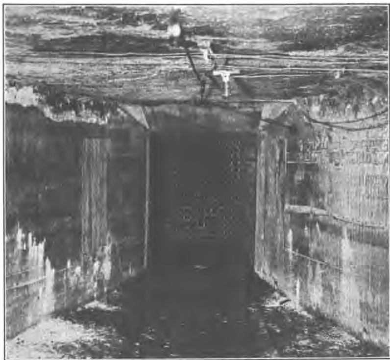
FIGURE 7.—General view of departure side of 1B-100 air-measuring station
