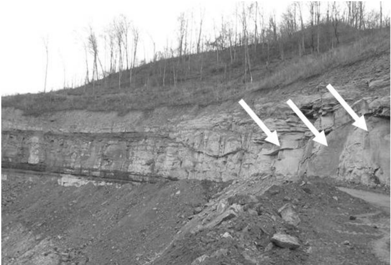
Figure 8. Web pillar failure occurred along highwall to the right. Note that several large rock wedges were dislodged as indicated by arrows. Undamaged highwall is to the left.
