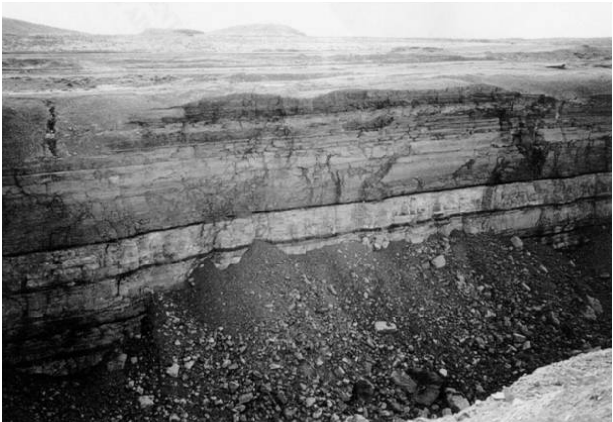
Figure 9. Site of massive web pillar collapse resulting in highwall slope failure. Photograph is taken from adjacent spoil pile. Highwall is about 150 feet high. A 110 ton coal haulage truck is buried in rockfall debris.
