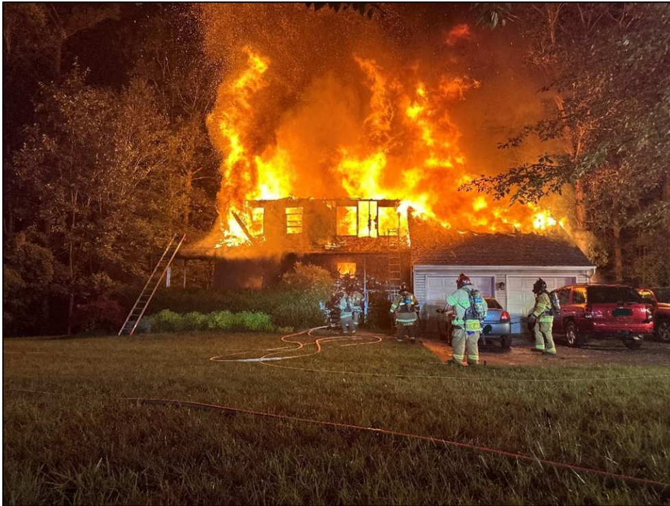
Photo 4. Fire conditions after second floor collapse (Courtesy of Southern ScanMD.org)
