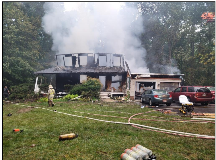
A view of the structure from side Alpha after the fire was knocked down.
