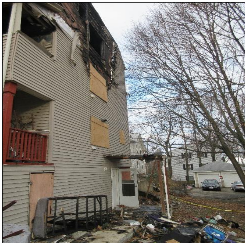
3 rd floor porch window Ladder 5 firefighter went out of and initially landed on awning over basement door. (NIOSH Photo)
