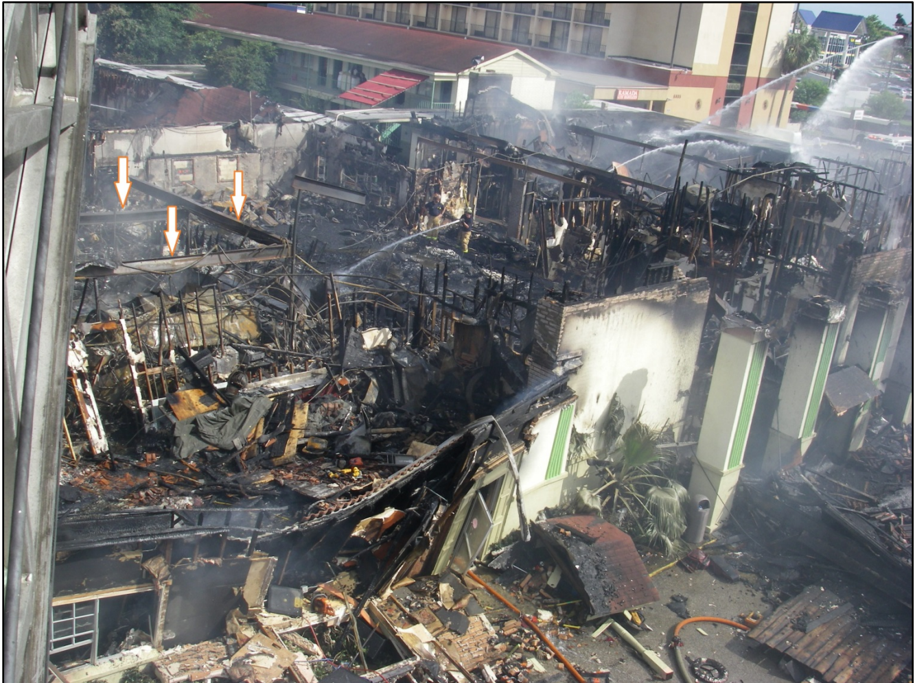
Photo 4. The arrows indicate the support system for the 2 nd floor and void space above the restaurant and lobby area of the motel.
