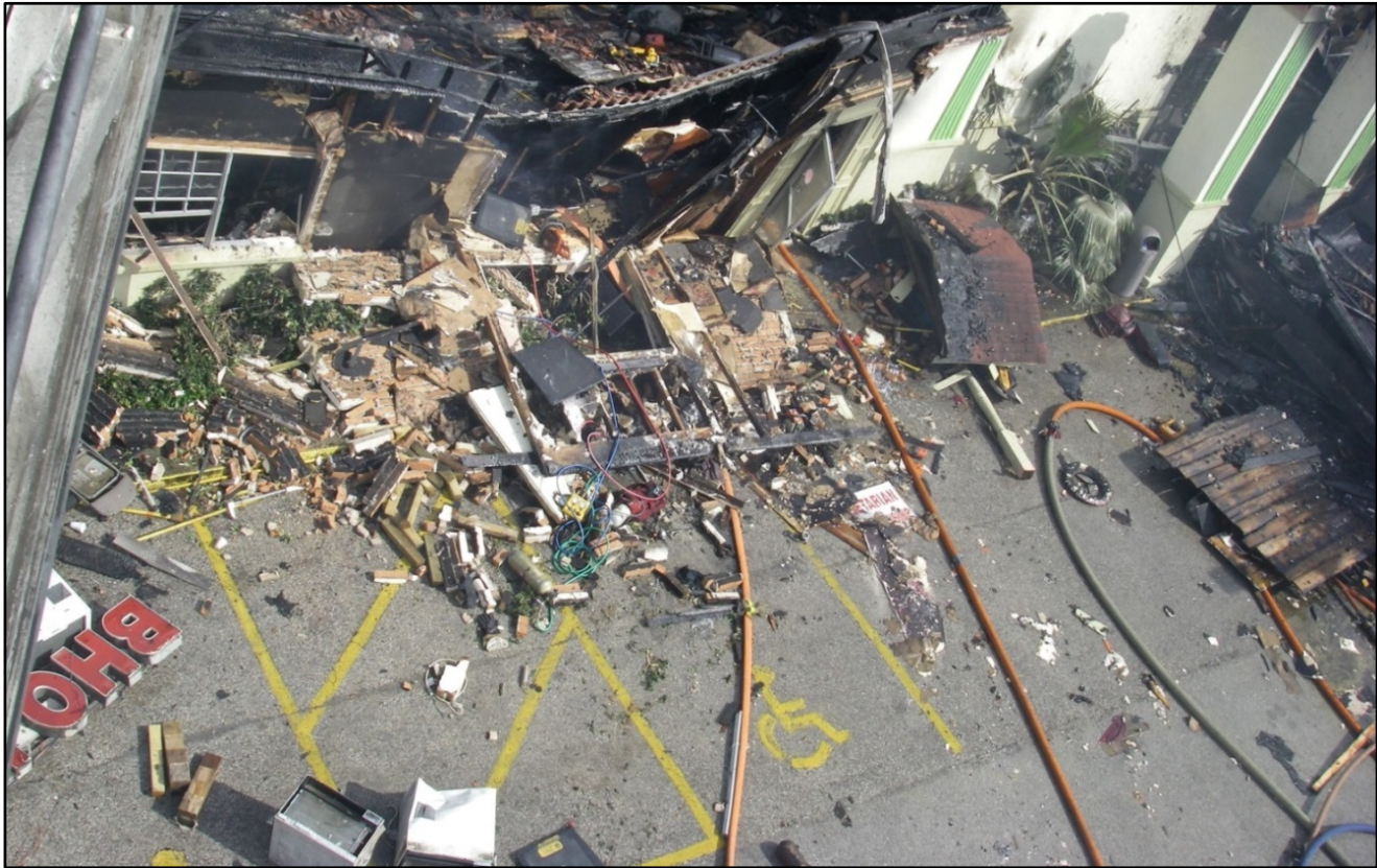
Photo 7. The front façade collapsed at 1303 hours striking fire fighters and officers assigned to the Rescue Group. These members were quickly removed by other fire fighters who picked up the façade and pulled the trapped fire fighters and officers out. (Photo courtesy of the fire department)
