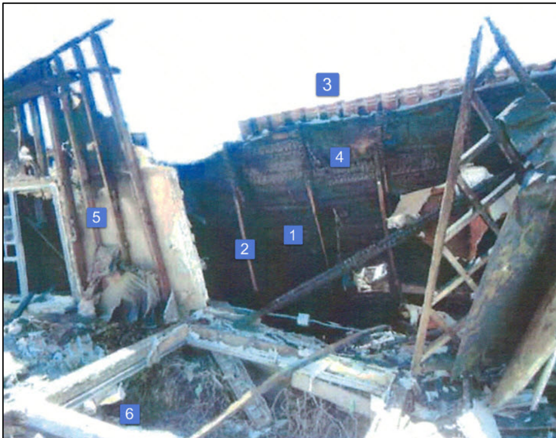
Photo 1. View of Division Alpha Perimeter Wall & Lean-To Roof Collapse (Fire Department Photo/ Diagram Courtesy of Buildingsonfire.com)
