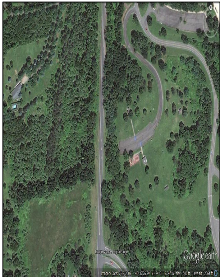
Aerial view of section of roadway where incident occurred.
