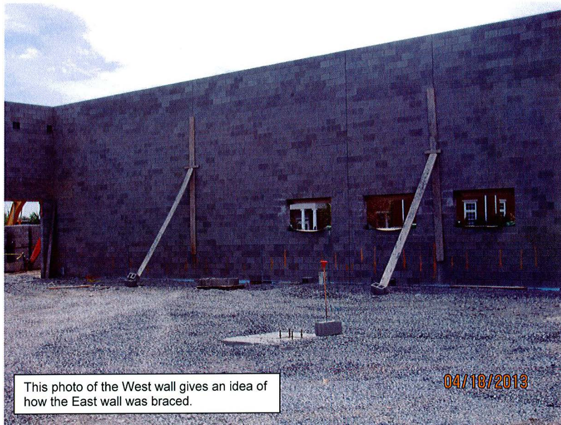
Photo 3. Interior wall bracing. (Photo courtesy of TOSHA.)
