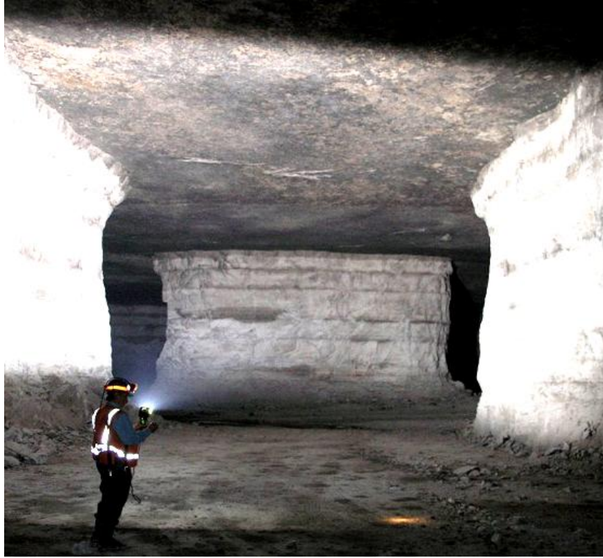
Figure 27. Naturally stable 13.4-m (44-ft) wide roof span in a stone mine.
