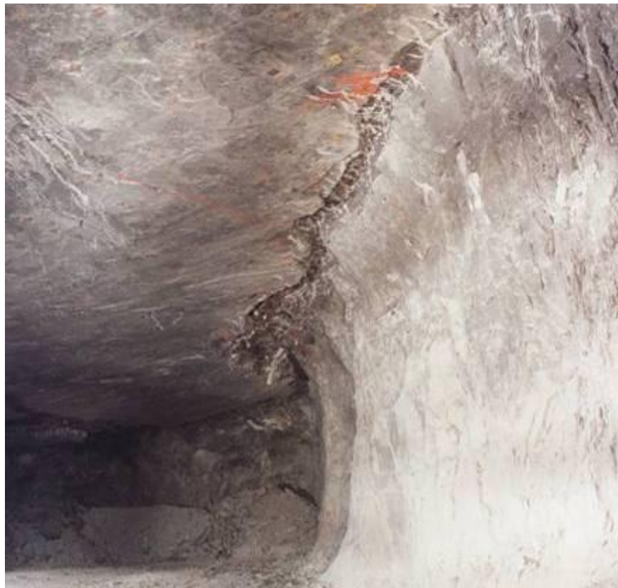
Figure 31. Roof guttering at the pillar-roof contact.
