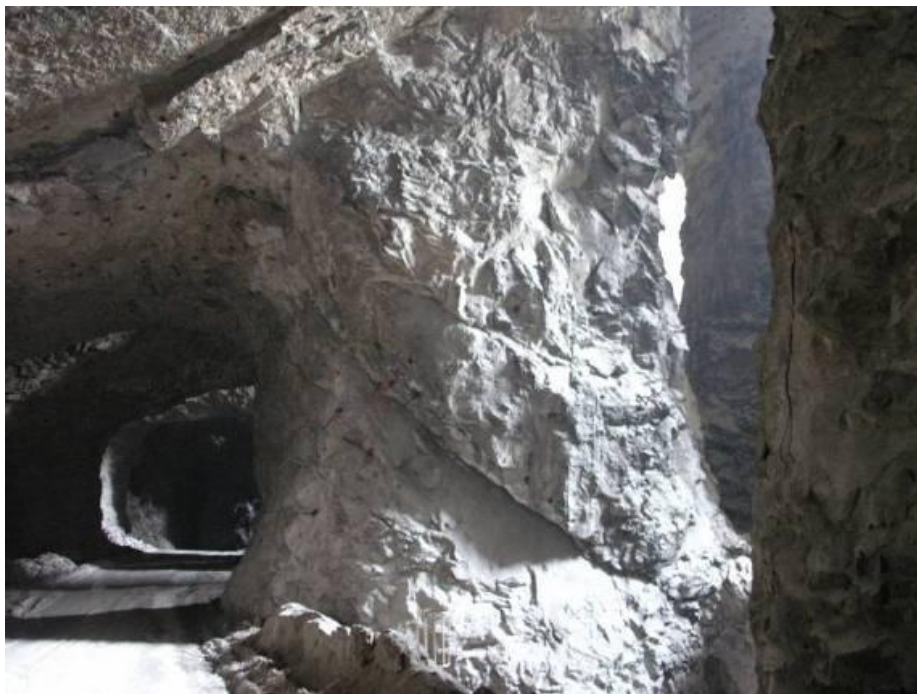
Figure 13. Example of a pillar that is bisected by a large, angular discontinuity.
