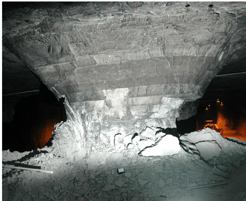
Figure 5. Pillar that had an original width-to-height ratio of 1.7, but failed by progressive spalling. Thin, weak beds are thought to have contributed to the failure. The average pillar stress was about 11% of the UCS prior to failure.
