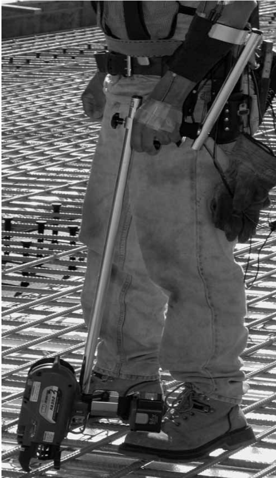
Figure 3. Rebar tying using a MAX-USA RB-392 power tool with adjustable extension.
